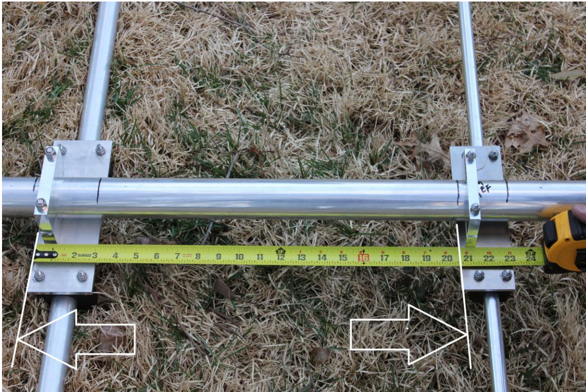
Figure 22 – Most effective way to measure element spacing. Always measure from the edge of the plate element #1 (20 Meter Reflector) to the element you are positioning on the boom. Use the leading edge of both plates. Do not measure the spacing element to element, as this accumulates inaccuracies
